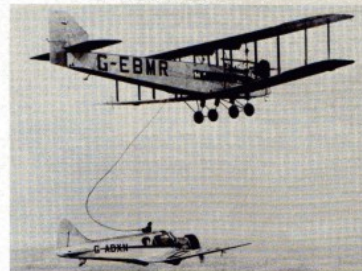
A Handley Page W10 was used by Cobham to refuel his Airspeed Courier in an attempt to fly non-stop to Australia. FRL
