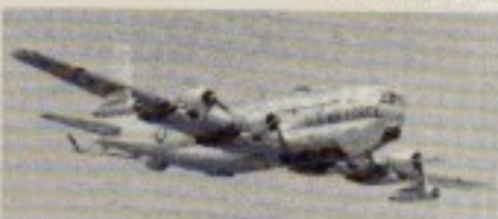
The flying boom system was adopted by the USAF in 1950, as fitted to this KC-97. PRM
